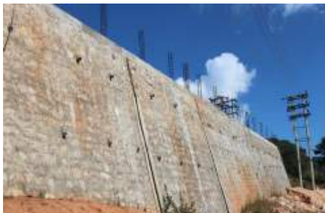
Plate 5.11: Retaining wall at 33/11kV Mawpat
