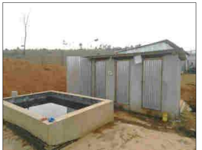
Toilet facilities at 220 kV New Shillong SS
