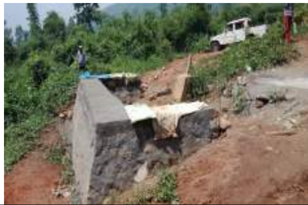
Plate- 5.13 Construction of Revetment Wall and ULE at AP 23/0 & 59/0 of 220 kV D/c Byrnihat-Mawngap-New Shillong line
