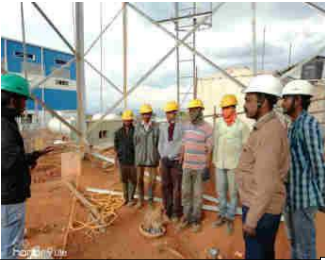
Height work training at Mawngap GIS Substation
