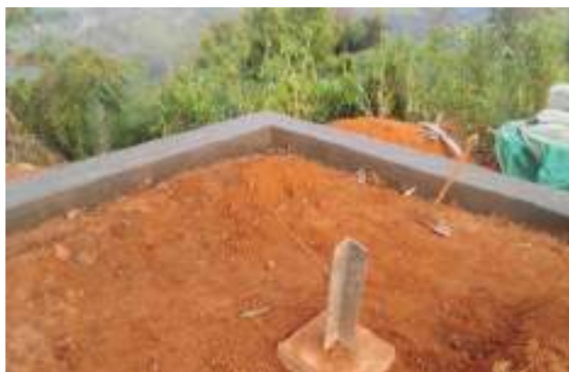
Plate- 5.13 Construction of Revetment Wall and ULE at AP 23/0 & 59/0 of 220 kV D/c Byrnihat-Mawngap-New Shillong line
