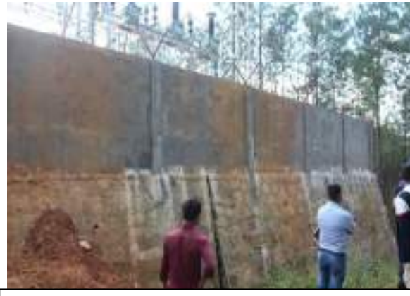
Plate 5.12: Retaining wall at 33/11kV New Shillong
